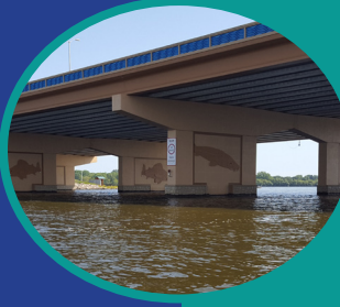
21 TRIBAL HERITAGE CROSSING BRIDGE
